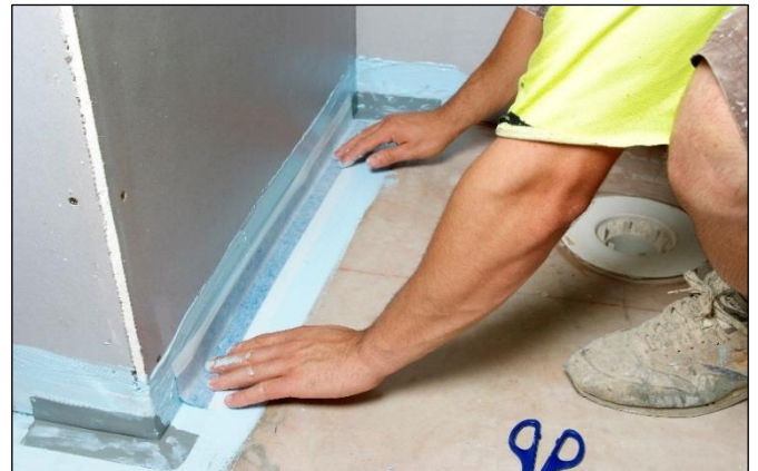
Installing Elastoproof B50 Bond Breaker Joint Band
