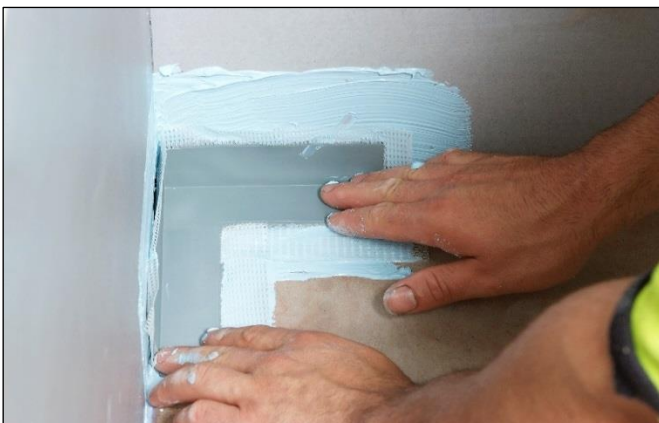
Installing Elastoproof Prefabricated Corners
