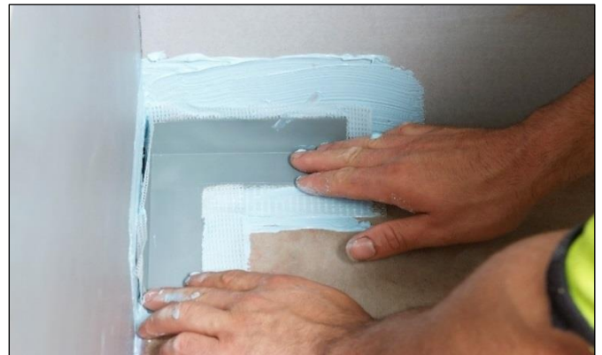
Installing Elastoproof Prefabricated Corners
