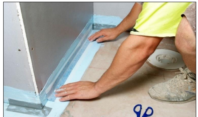
Installing Elastoproof B50 Bond Breaker Joint Band
